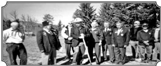
On Saturday, April 4, 2009, the first shovel of sod was turned by Shuswap M.L.A. George Abbott starting the construction of their new hall.
